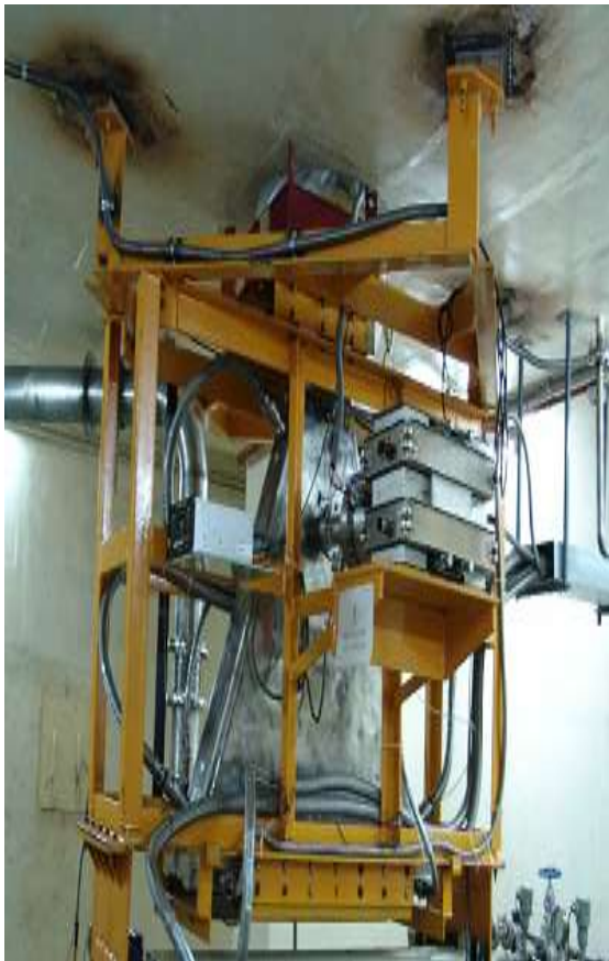
Ground Floor Scan Horn View
