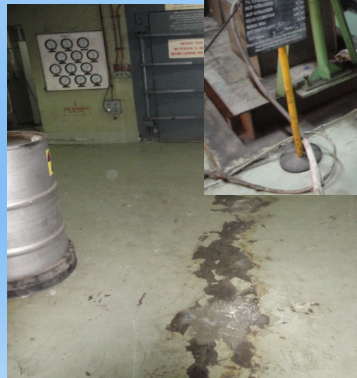
Sub-Soil Seepage in RCC RAFT/Joints
