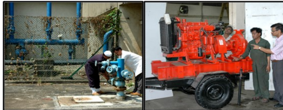
FIGURE SHOWING ECW LINE MODIFICATION WITH TROLLEY MOUNTED PUMP TO PUMP BACK UGDT WATER BACK TO OHST IN CASE OF EMERGENCY
