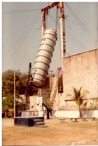
Fig. 4 (i): Installation stages of Pelletron
