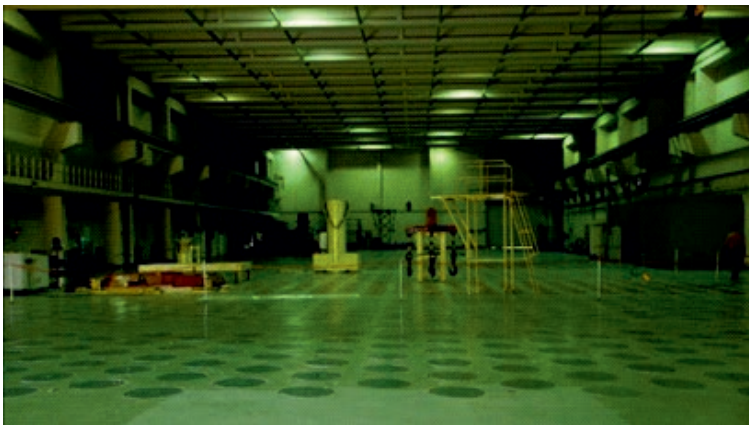
Solid Storage Surveillance Facility, Tarapur
