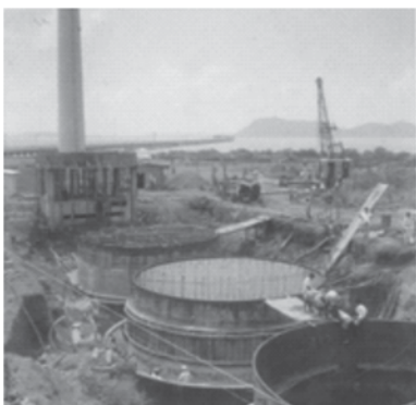
Construction of Low level tanks at ETP (Year 1962)
