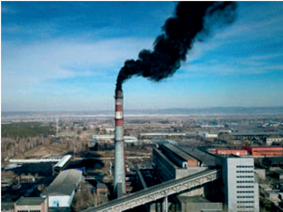
Fig. 2(a): A typical coal fired thermal power station. A typical 500 MWe coal fired unit releases about 10000 tonnes per day of CO 2 , which has major bearing on green-house effect. In addition, copious amount of So 2 , NOX gases and harmful Particulate Matter (PM) amongst others are also released. In the year 2021 India emitted about 1.4 billion tonnes of CO 2 owing to coal firing at power stations alone
