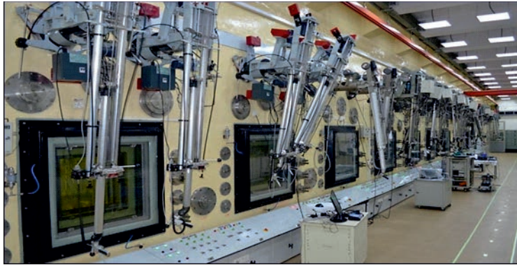
Fig. 15: PIE Hot Cell at BARC, for Metallurgical and Mechanical Studies on Irradiated Fuel and Reactor Core Materials such as Pressure Tubes of PHWRs. This is the Second Largest PIE Hot Cell in the world. It has 1.5 m thick concrete shielding and special Radiation Shielding Windows. Components having contact dose rate up to about 30000 R/h have been successfully handled in these hot cells
