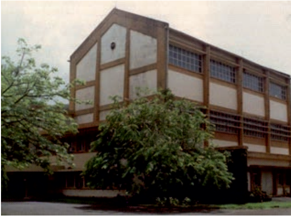
Fig. 5(a): APSARA Reactor: Outer View of Reactor Building. Fuel and Pool Details shown in Fig.6(a) and Fig. 6(b). (Operations started in the year 1956)
