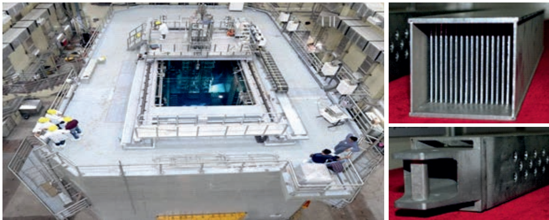
Fig. 13: Left Picture- APSARA-U reactor pool in operation. Bluish glow owing to Cherenkov radiation is seen. Right Pictures- APSARA-U fuel assembly Cut-away View and Full View. Uranium silicide fuel, for ASARA-U, is first of a kind in India
