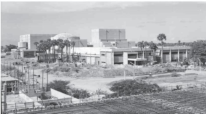
FBTR after completion of civil construction, 1977
