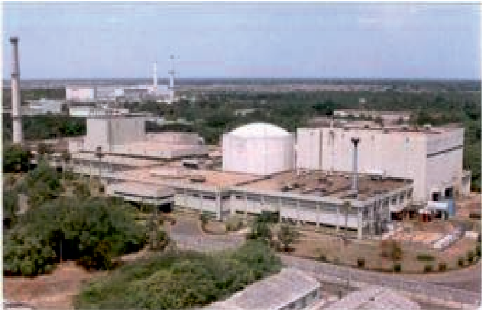
Fast Breeder Test Reactor
