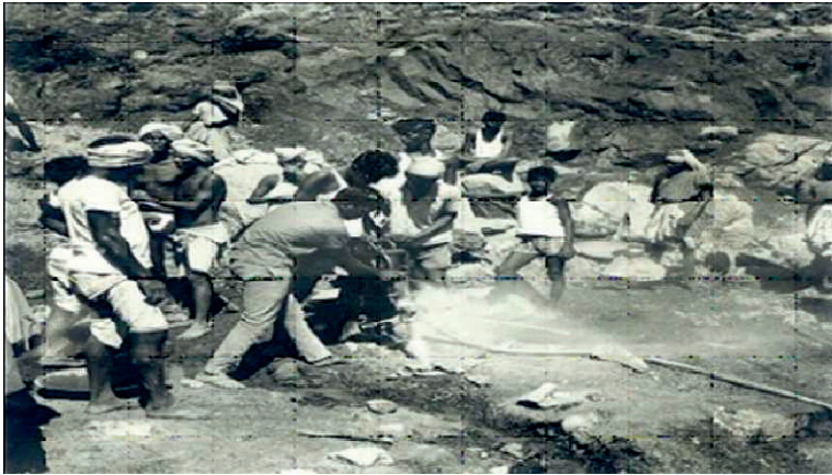
Rock Breaking activity at Fast Breeder Test Reactor construction site
