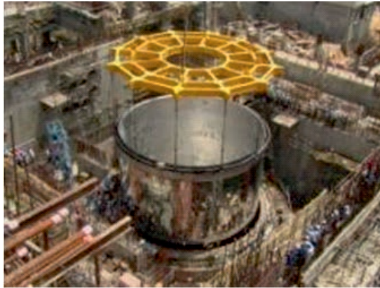
Lowering of Safety Vessel in reactor vault
