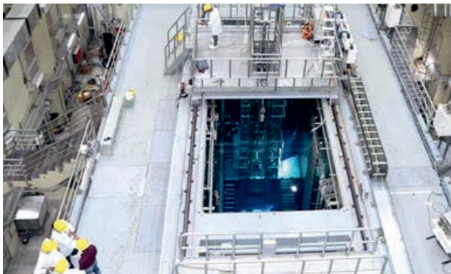
Reactor Pool of Apsara-U Research Reactor at BARC
