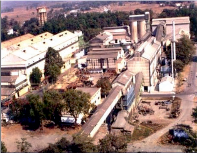
Fig.8: Aerial view of Jaduguda Processing Plant
