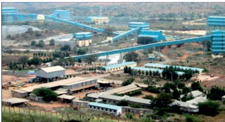
Fig.11: Aerial View of Tummalapalle Processing Plant
