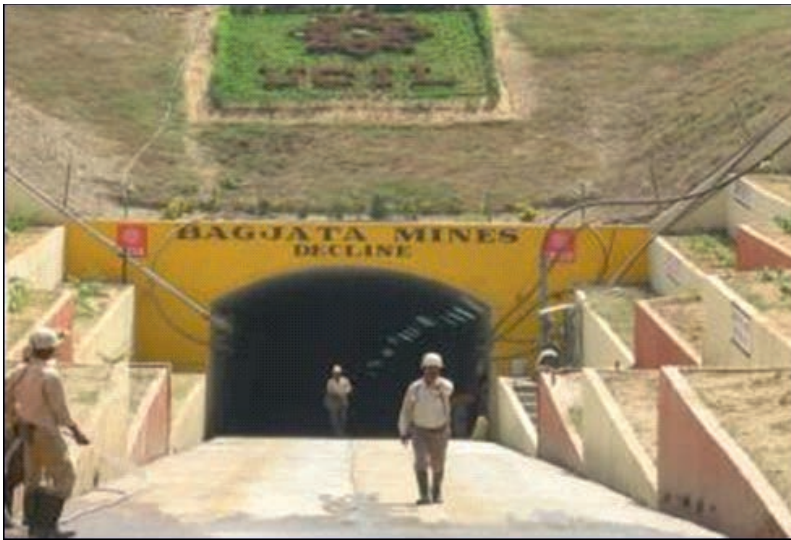
Fig.6: Decline Entry of Bagjata Mine
