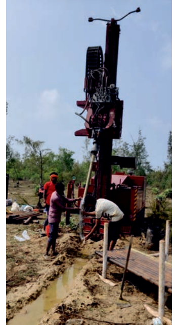
Fig. 11: Sonic Drilling in Beach sands of Brammagiri area, Puri district, Odisha
