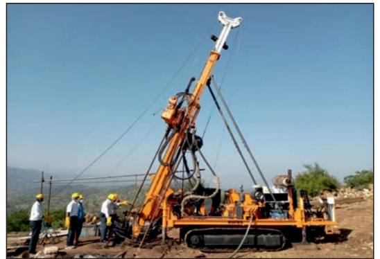
Fig. 5: Sub surface exploration for uranium by crawler mounted hydrostatic drilling rig
