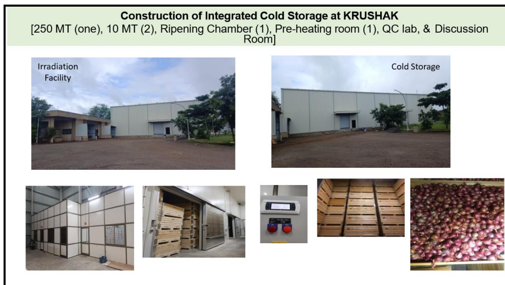
Fig. 4: Onion specific cold storage facility for technology demonstration commissioned at KRUSHAK, Lasalgaon
