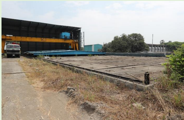
Reinforced Concrete Trenches (RCT)
