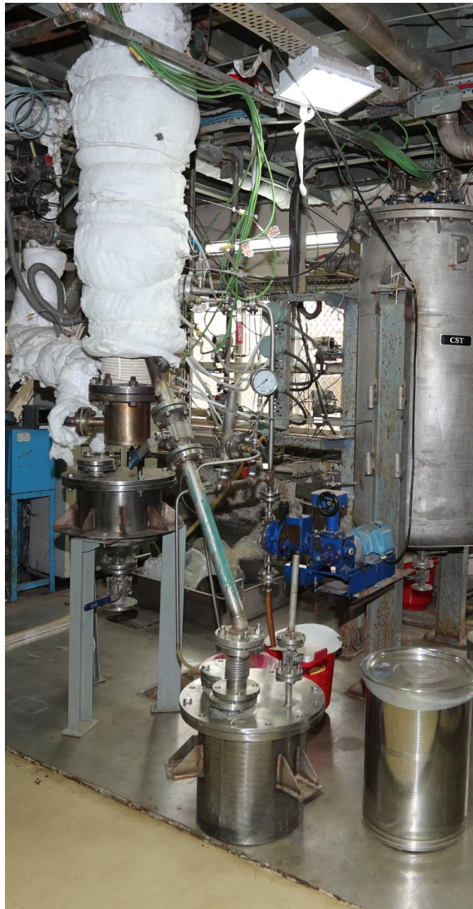
Bench Scale Denitration Facility at CEL – 3, ChED
