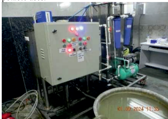
Kitchen waste water treatment skid in operation in BARC.
