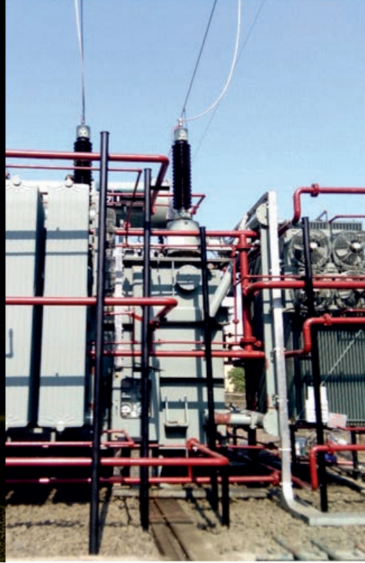
50 MVA Transformer (TF-2) commissioned in BARC Trombay.
