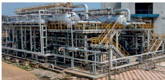
2 x 250 m 3 /d MED-TVC Desalination Plant at IREL, OSCOM.
