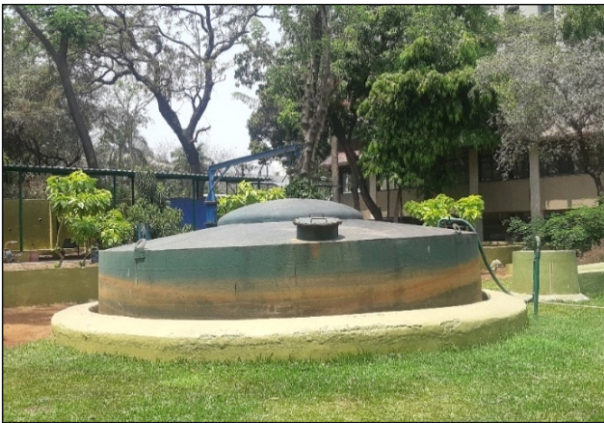
Fig.2: Nisargruna plant at Trining School Hostel, Anushaktinagar.
