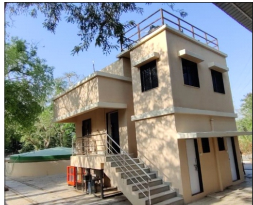
Fig.3: Nisargruna plant at BARC Hospital, Anushaktinagar.
