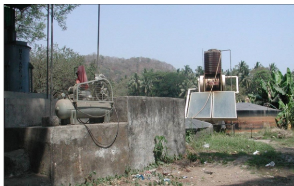
Photo.1: First Nisargruna plant installed at Nursery, BARC 2001.
