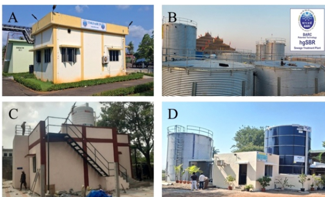
Fig.3: Photographs of some hgSBR-STPs. A) 1500 m 3 /day plant at Kalpakkam township. B) 500 m 3 /day plant used during Maha Kumbh 2025 at Prayagraj. C) 150 m 3 /day plant at Surat. D) 400 m 3 /day plant at Sangmaner.
