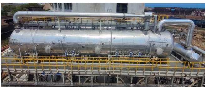
The Seawater reverse osmosis plant established by BARC at OSCOM in Odisha.
