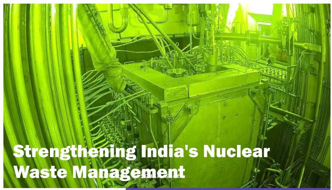
The Joule Heated Ceramic Melter (JHCM) in operation at AVS Annex Facility in NRB Tarapur.
