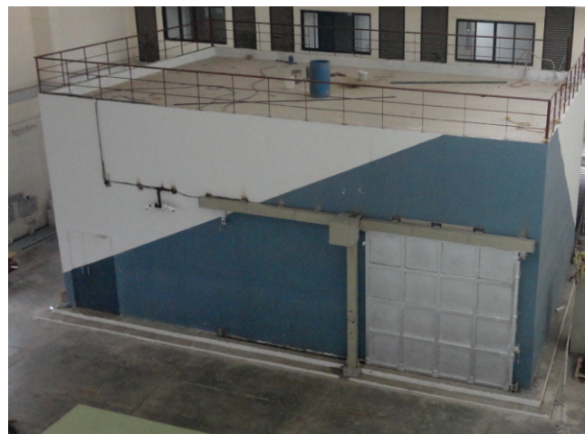
Fig.2: Newly built hall exclusively for the ECRIS at Hall-9, BARC.
