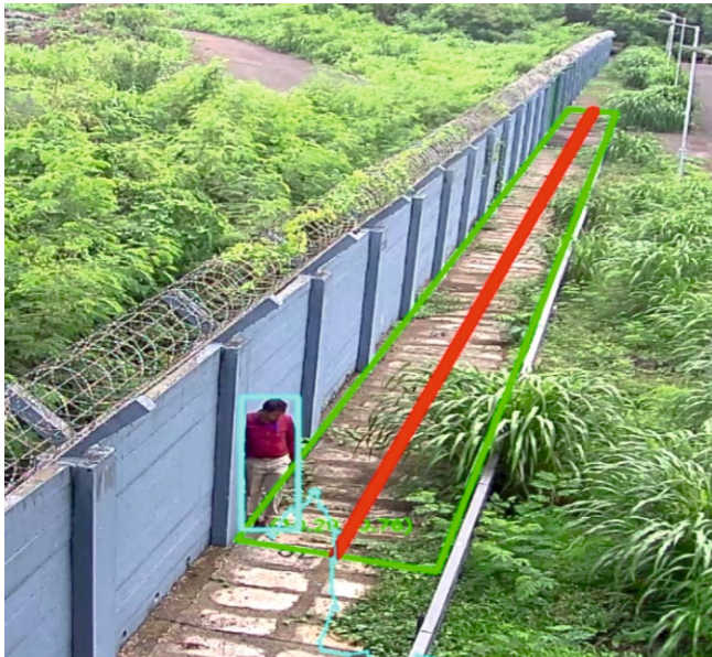
Fig.4: Zones are marked up to 50m. Red line is virtual fence and green is zone. It detects persons and tracks them. As soon as the person enter the zone, a bounding box is drawn around him and the tracking of the movement is performed.
