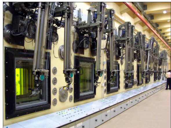
Fig.5: A row of RDMs installed in hotcell.
