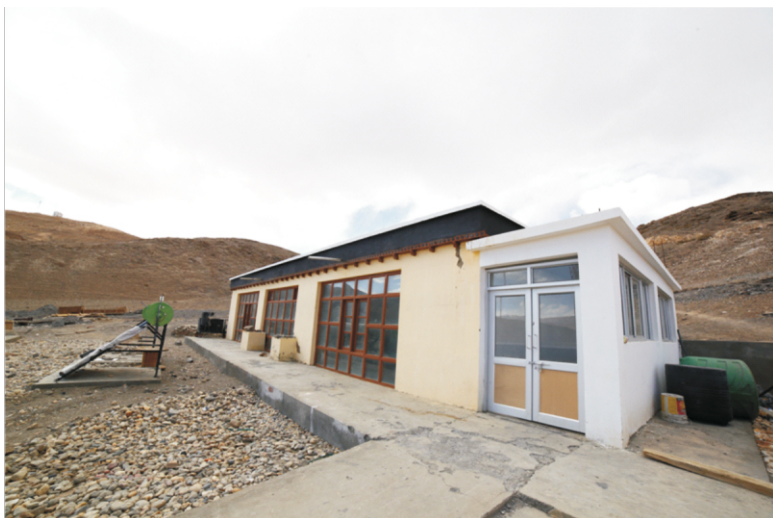
▲ MACE control room facility situated at Hanle site.
