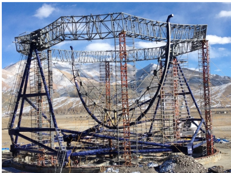
▲ THE ASSEMBLY of the alidade structure with stiffening ring and bull-gear support structure of the telescope was completed at Hanle in November 2015.
