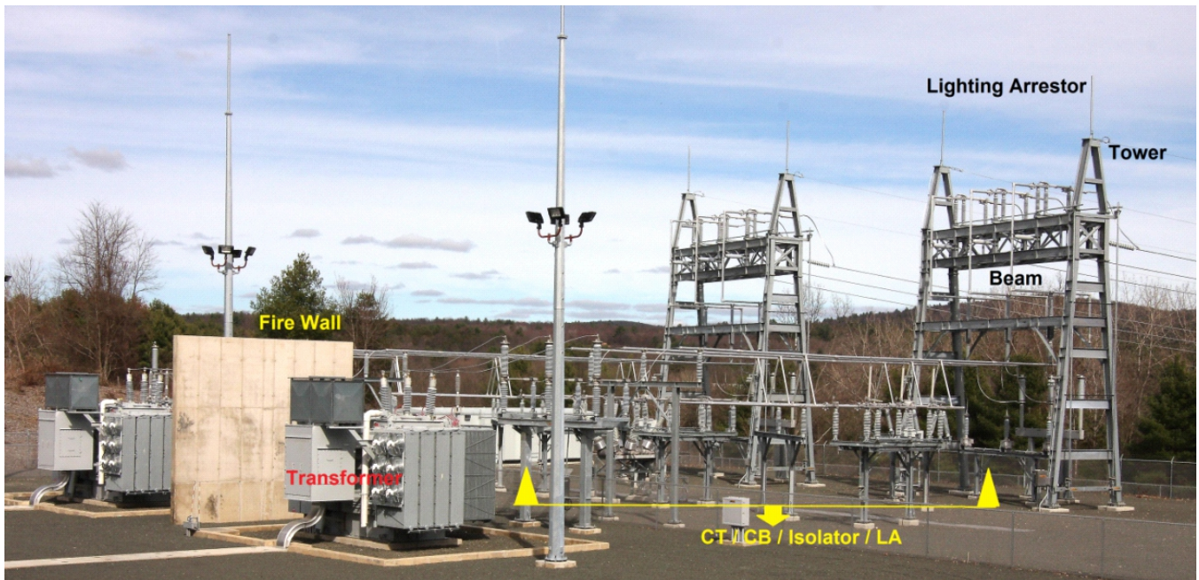
Fig.1: Some components of a typical electrical substation.
