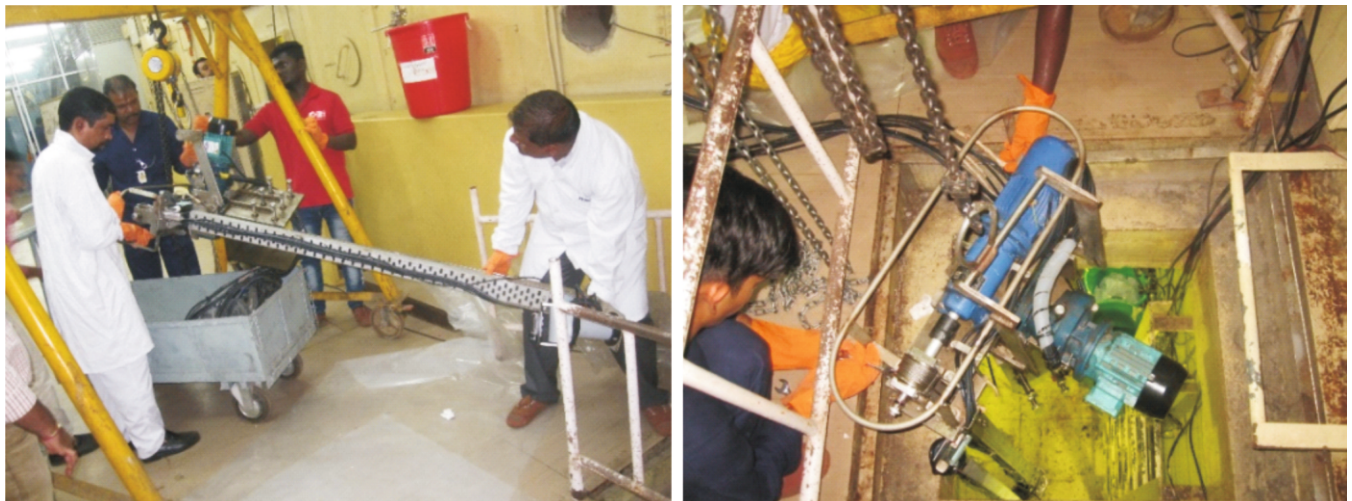
Fig.5: Shifting and insertion of assembly inside the cell.
