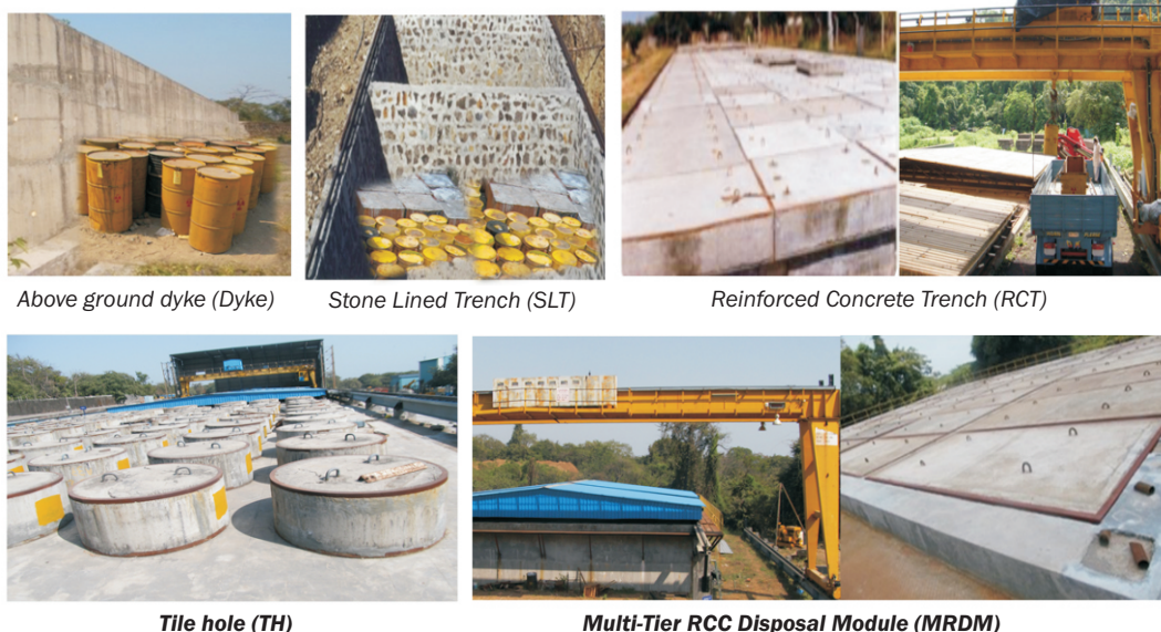
Fig.1: Typical Engineered disposal modules of Near Surface Disposal Facility.
