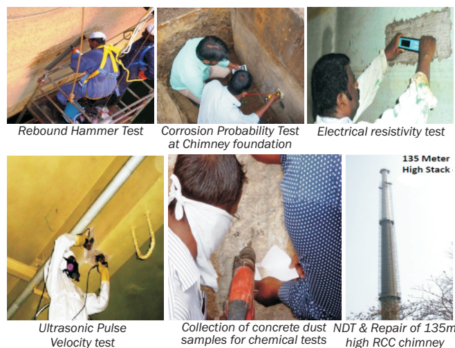
Fig.5: NDTs of different structures in NRG facilities.
