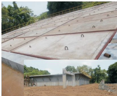
Fig.3: Multitier Reinforced Concrete Disposal Module at RSMS, Trombay.
