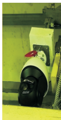
Fig.11: Remotely replaceable wireless camera system.
