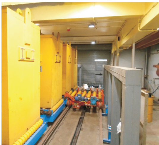
Fig.3: Self-shielded Ion Exchange columns.
