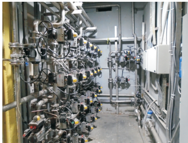
Fig.4: Valving station of Ion Exchange system.
