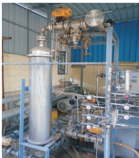
Fig.5: Ultrafiltration Pilot Plant.
