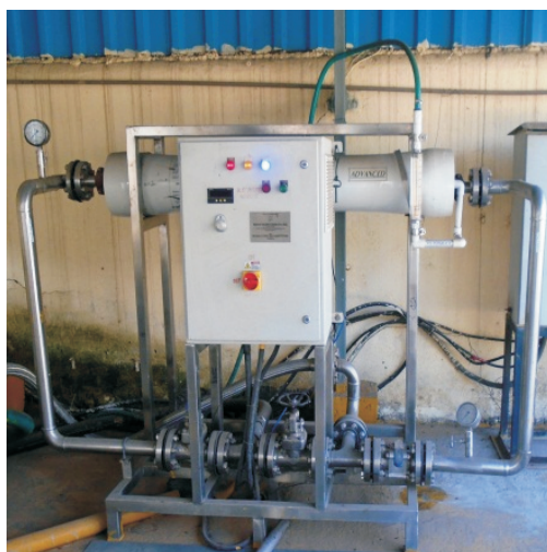
Fig.6: Spiral RO Pilot Plant.
