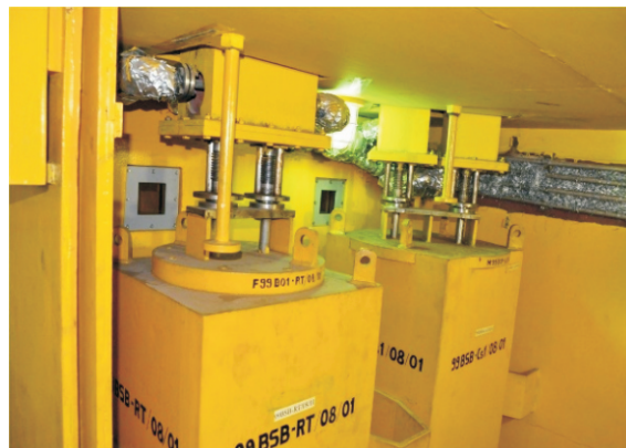
Fig.4: Incell view of Ion Exchange system.
