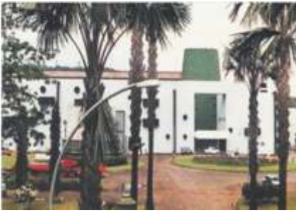
Fig.2: Reprocessing Plant, Trombay.
