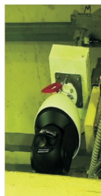
Fig.11: Remotely replaceable wireless camera system.
