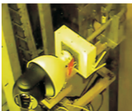
Fig.10: Wireless camera on cell crane.
