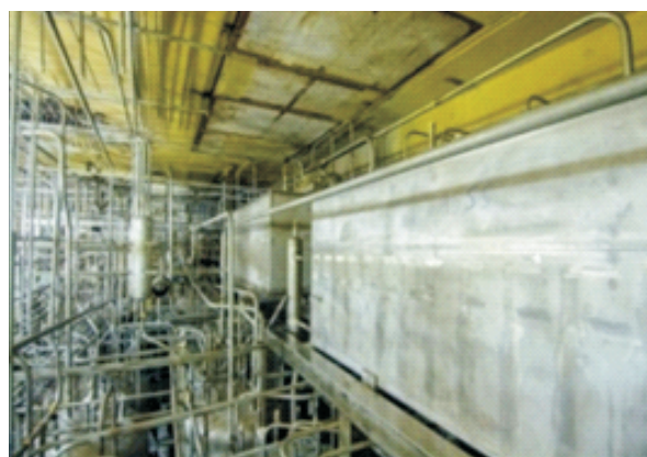
Fig.2: Solvent extraction system, Trombay.
