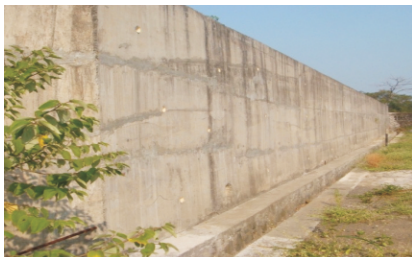
Fig.2: RCC dyke at RSMS Trombay.
