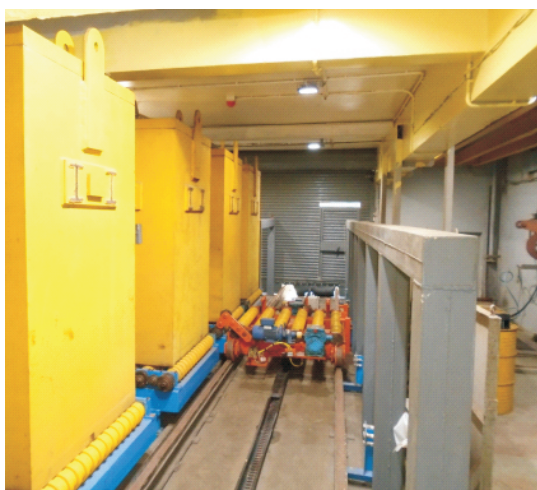
Fig.3: Self-shielded Ion Exchange columns.
