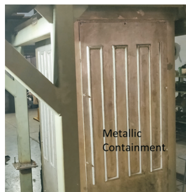
Fig.4: Secondary metallic enclosure.
