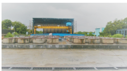
Fig.4: Tile Hole Battery at RSMS, Trombay.
