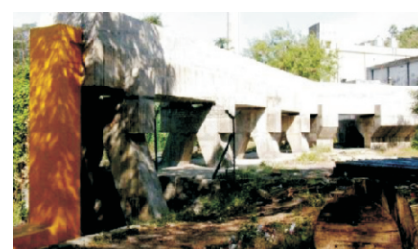
Fig.1: Above ground RCC HLW Transfer Duct from AWTF to WIP Pump House.
