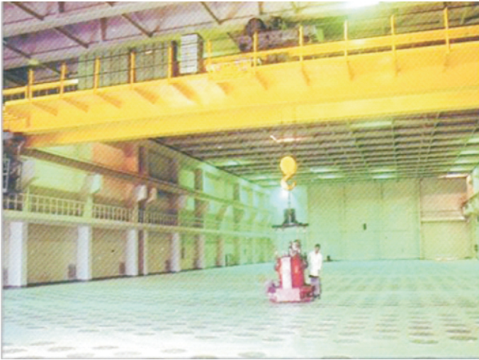
Fig. 2: Solid Storage and Surveillance Facility at Tarapur
