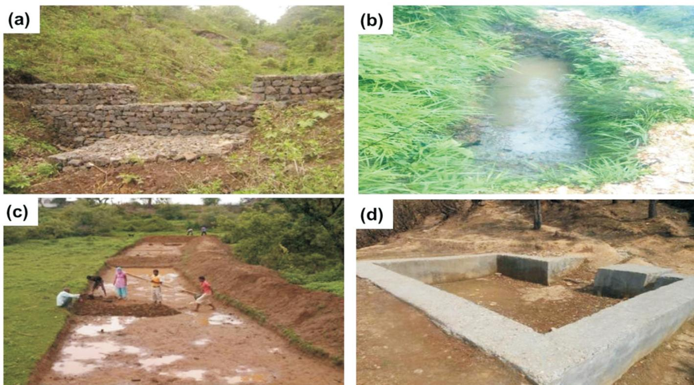
**Fig.6:various recharge structures constructed at the identified recharge zones, a) gabion check dam, b) infiltration pits, c) contour bunding and d) percolation ponds**
