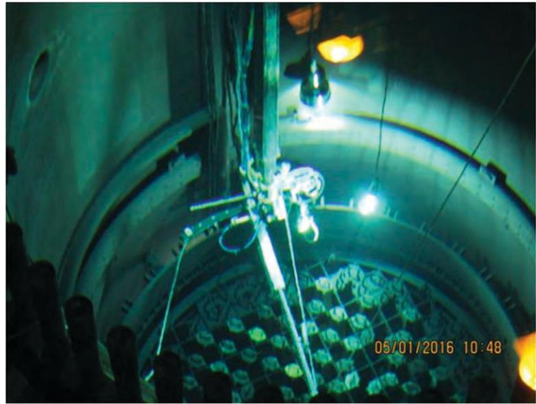
Fig. 23: Performing Weld Inspection
