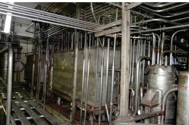
The mixer-settlers with passive mixing devices located inside the radiological cell
