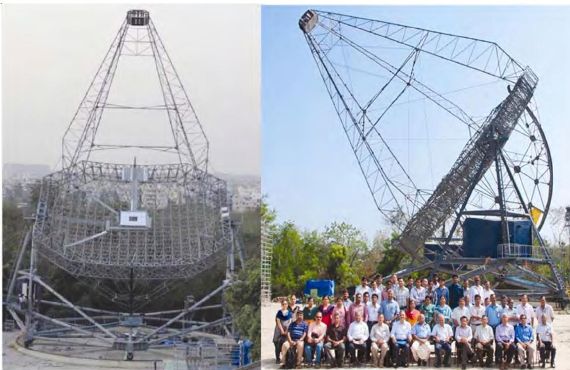
The picture on the left shows 8 mirror panels installed around the centre of the mirror basket. The servo TDU and TCU are installed in the instrumentation shelter mounted on the adelaide structure. The picture on the right shows the participants of the CDR meeting gathered in front of the proof-assembly
