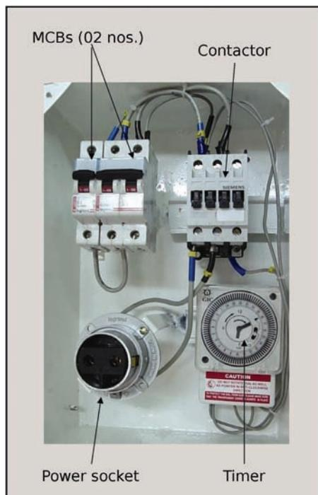
Fig. 3: Timer Control Device
