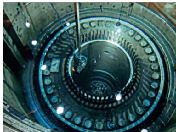
Fig. 15: WIM performing weld cleaning
