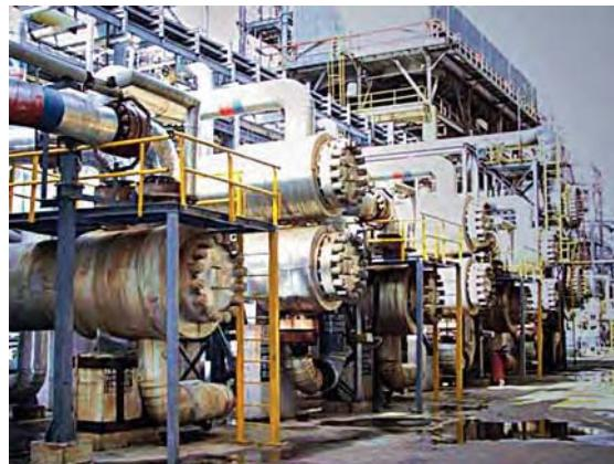
Fig. 5: A typical heat exchanger system in a refinery
