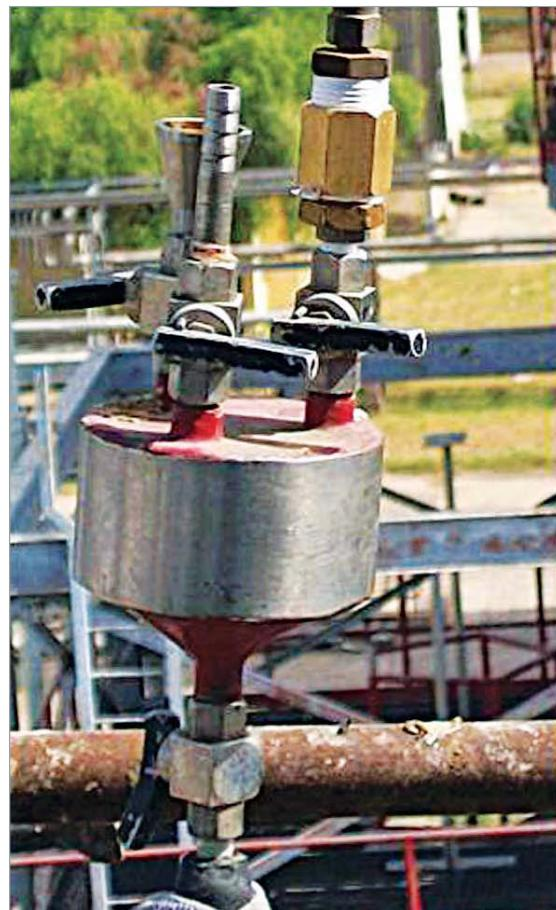
Fig. 2: A typical tracer injection system
