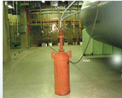
Fig. 2: A view of filter column connected to liquid waste storage tank during plant scale decontamination
