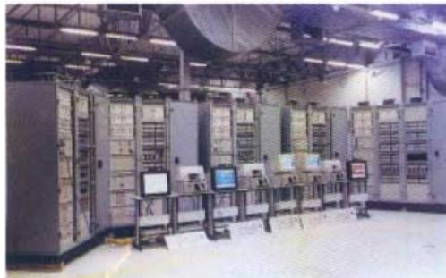
*Overview of SCADA hardware showing (from left) panels for RAPP-4 Turbine Building, RAPP-3 Turbine Building, RAPP-3 Control Equipment Room, RAPP-4 Control Equipment Room and the RAPP-3,4 Switchyard. In the foreground are the three Operator Display station computers and two server computers.*
