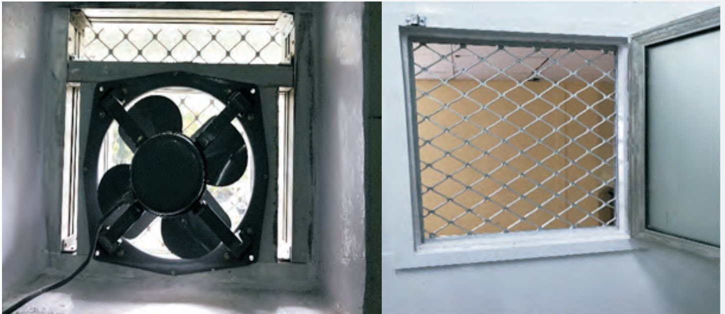
Fig. 2: Exhaust fan installation and ventilation port made in minor operation theatre
