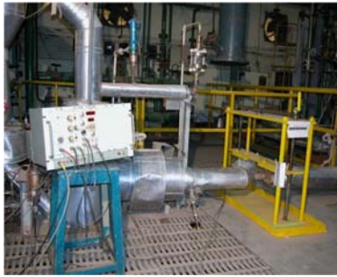
Steam-Water facility Expt
