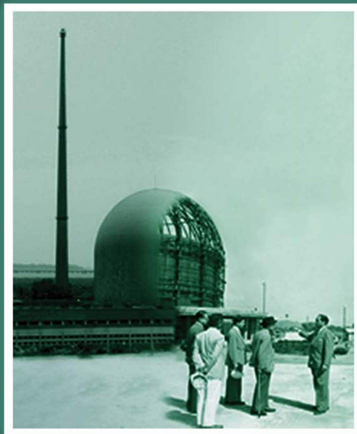
Dr. Homi J. Bhabha at the Cirus Construction site
