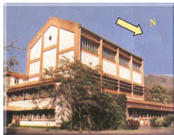
Fig. 9: View of APSARA reactor building
