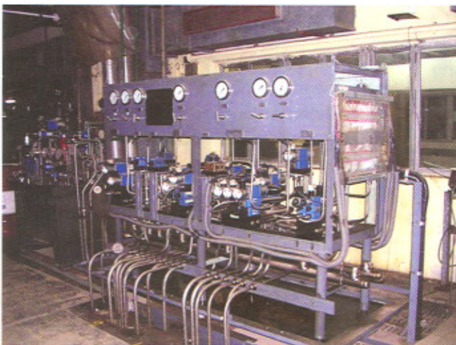
Fig. 3: Oil Hydraulic System of 540 MWe PHWR
