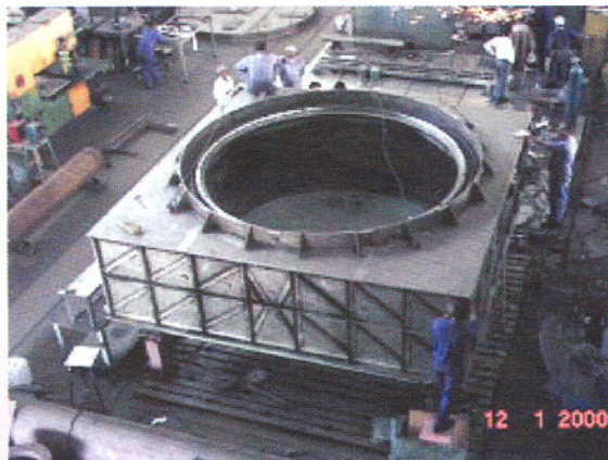
Fig. 3: Fabricated square box
