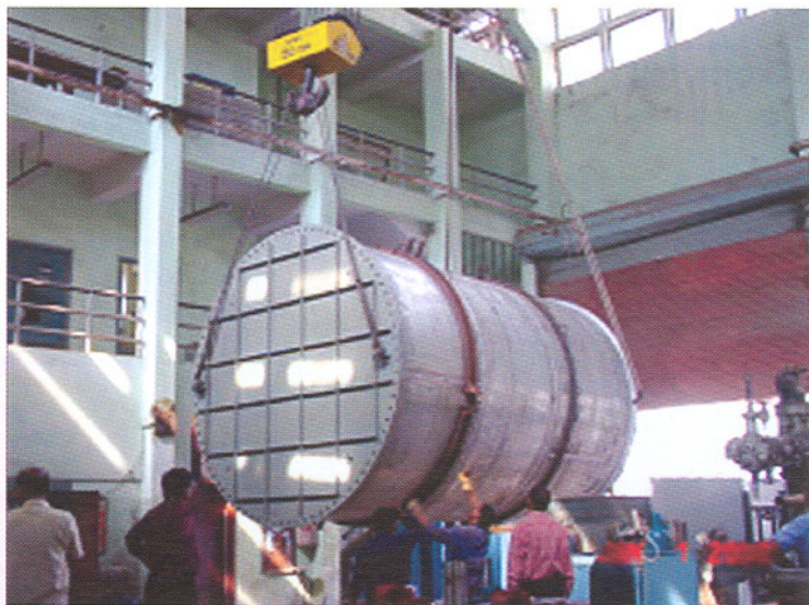
Fig. 2: Handling of Reactor Tank
