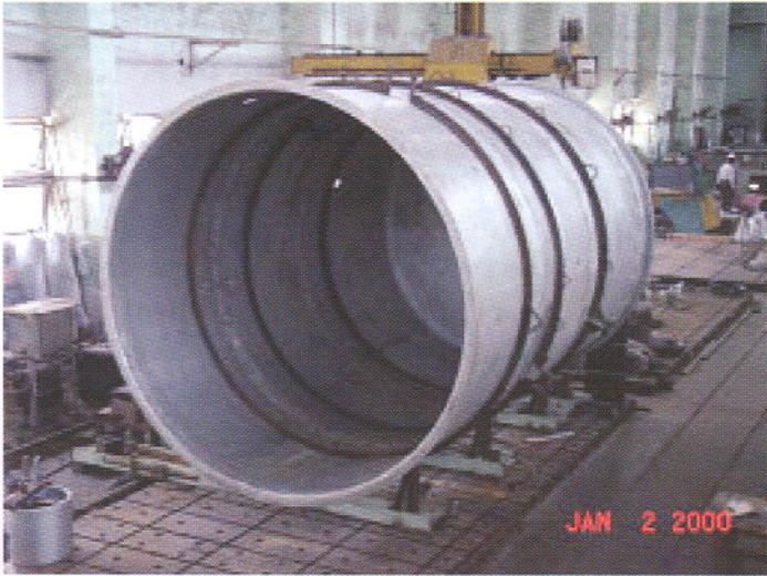
Fig. 1: Reactor Tank under fabrication
