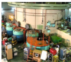
Neutron Scattering facilities in Dhruva reactor hall
