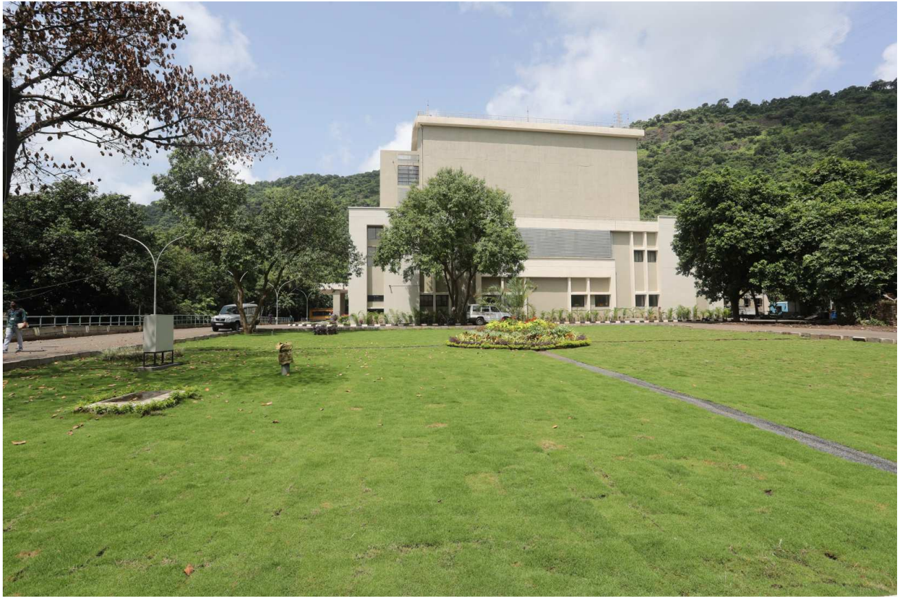
APSARA- U REACTOR COMPLEX
